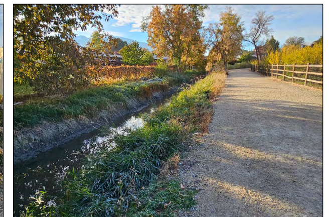
MAINTAINED TRAIL EDGES AND PAVING
