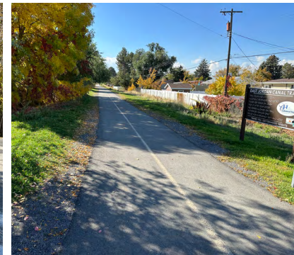
Existing EJCT over buried canal
