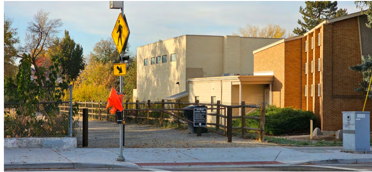
Rapid Flashing Beacon Crossing; Ada Ramps; Vehicle Access Gate; and Boundary Fencing (Post And Rail W/ Chainlink Infill)
