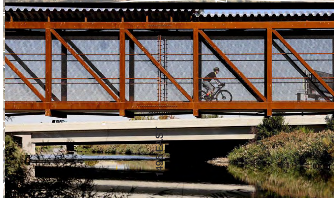
Box Truss Pedestrian/Bike Bridge (#1.1)
