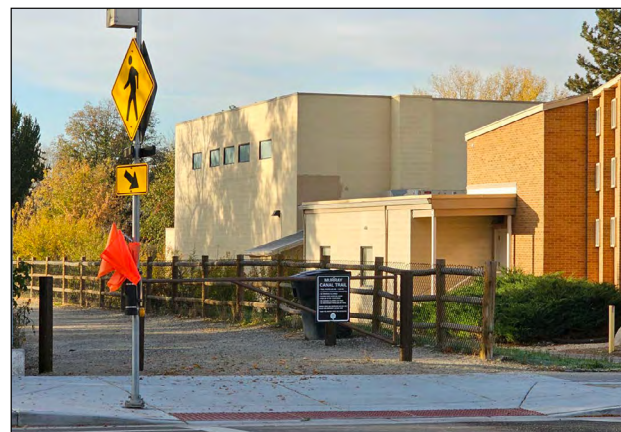
FLASHING BEACON CROSSING ADA RAMP VEHICLE ACCESS GATE BOUNDARY FENCING (POST AND RAIL W/ CHAIN-LINK INFILL)
