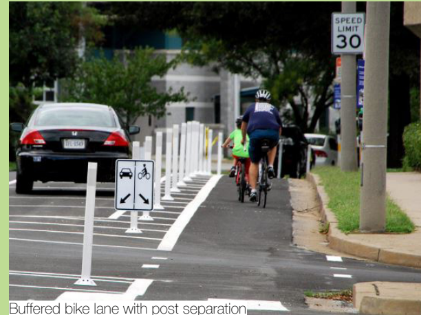
Buffered bike lane with post separation
