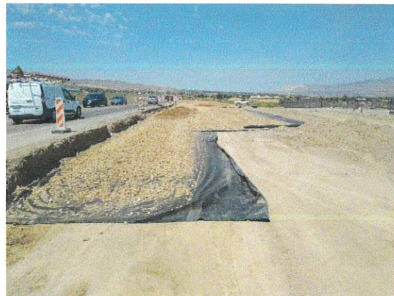
Saratoga Springs Foothill Blvd Construction Management Soft-Subgrade Mitigation
