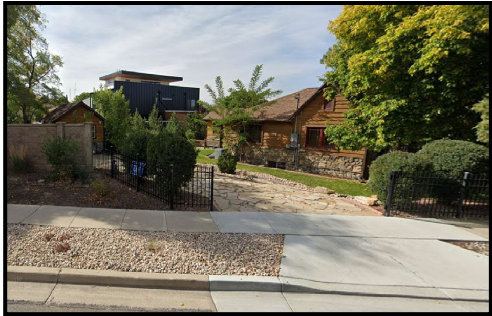
Subject Property Streetview
