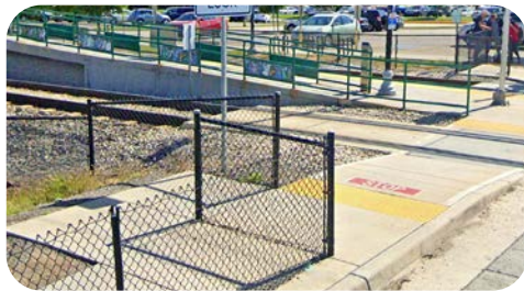
Figure 26. Chicane fencing are installed at places like rail crossings to increase safety by slowing down people on foot or bikes and to make them look both directions before crossing. Image source: Google
