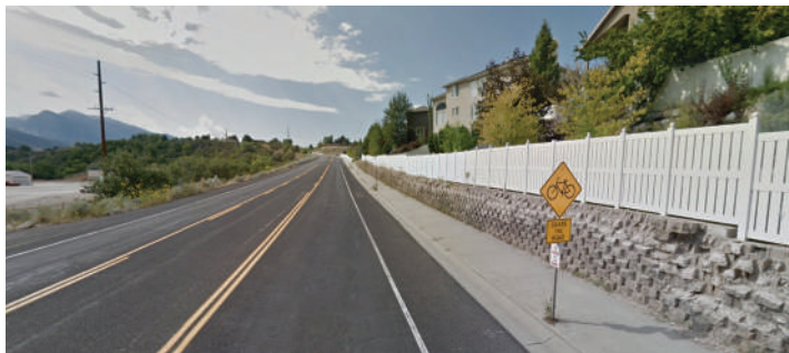
3000 South: from this image looking south the road reaches its maximum grade for light rail and streetcar, however, the slope is still within the acceptable range
