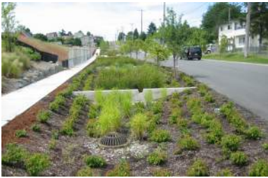
IDEA Bioswales: such as the example pictured here could improve the storm water runoff along the street
