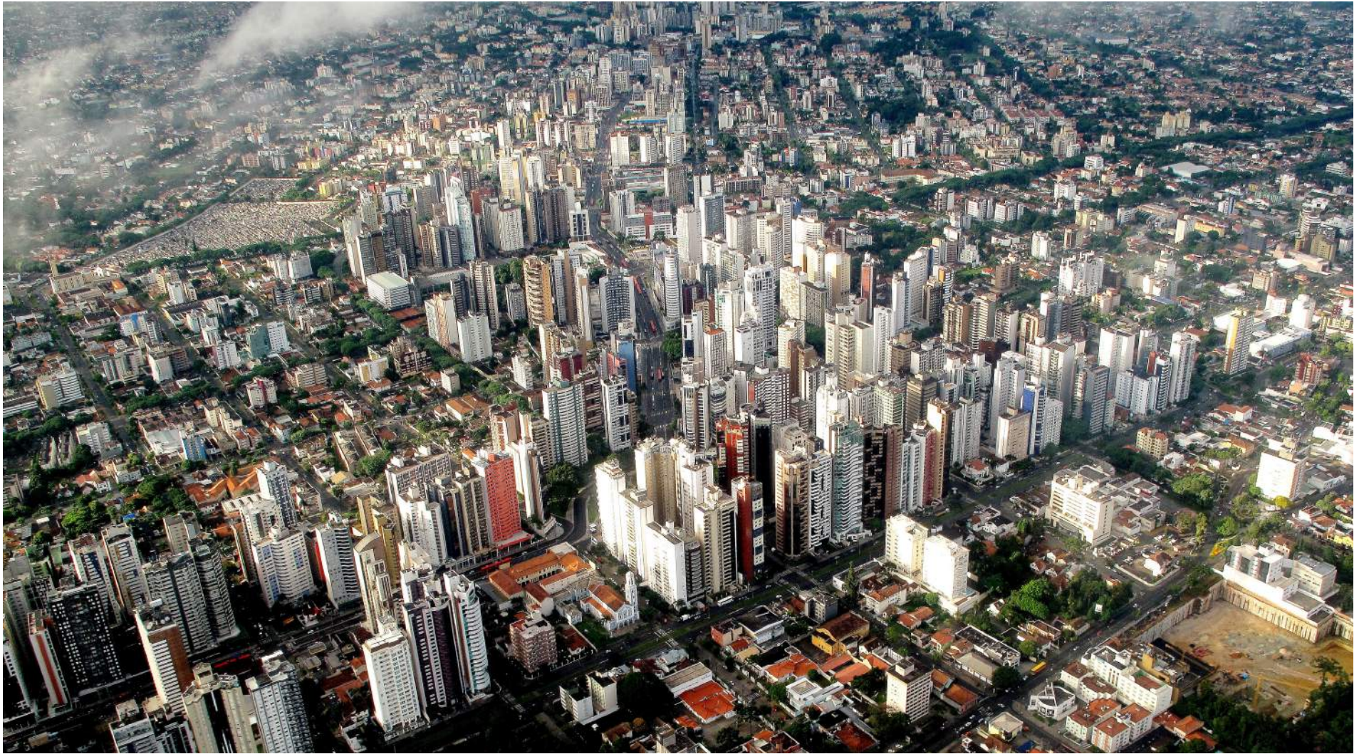
Curitiba, Brazil: the intersection of two bus rapid transit lines which has induced high density development around the lines
