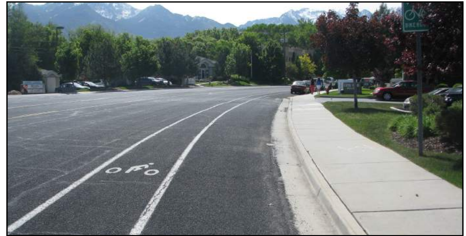
Creek Road, the boundary between Cottonwood Heights and Sandy, includes a Category 2 bicycle lane on both sides of the Road between Highland Drive and Union Park Avenue.
